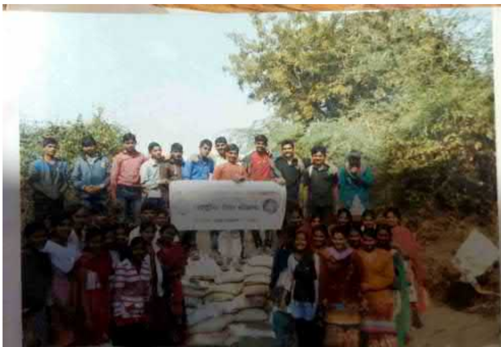
Making of “Vanrai Dam” at YawaliShahid under “Block the Water, Drain the Water” by N.S.S. Volunteers. Date : 13-02-2018
